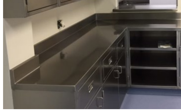
stainless steel countertops fabricated to drawings indicating backsplash height, raised edge and field condition requirements
