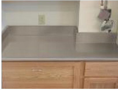
stainless steel countertops fabricated to specifications, indicating backsplash height, raised edge and field condition requirements
