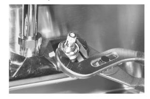
Step 3 - Remove the locknut with an adjustable wrench, then lift the spindle out of the faucet.
