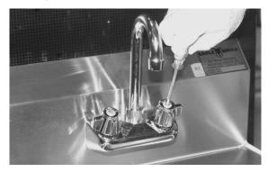
Step 2 - Remove housing retainer nut with a pair of channel lock pliers.
