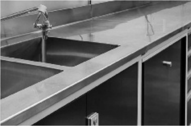
stainless steel countertops fabricated to drawings indicating backsplash height, raised edge and field condition requirements
